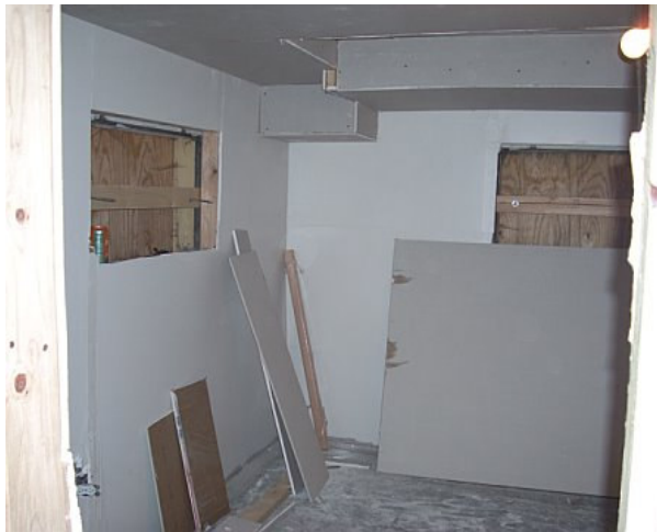
3rd BR in basement (This is now completed)
