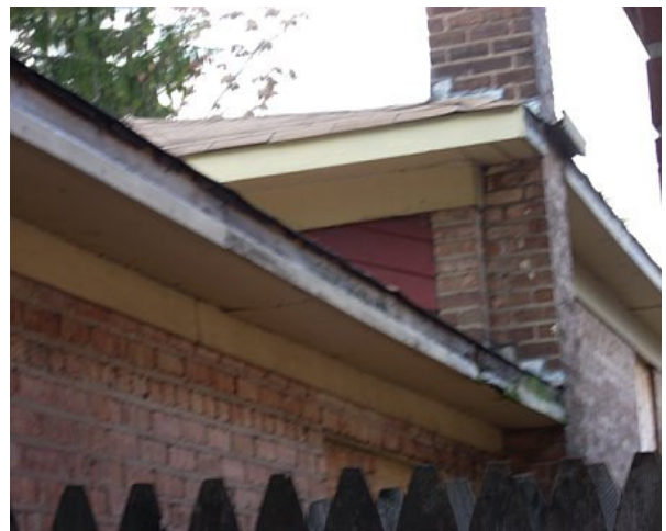
Check fascia on house
